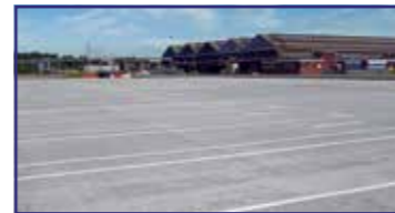
6,780 Tonnes Of Concrete!
