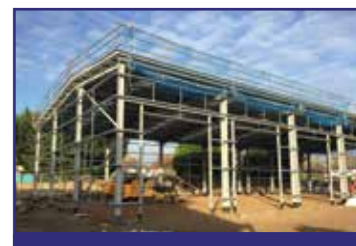
The New 47m x 19m Structure
