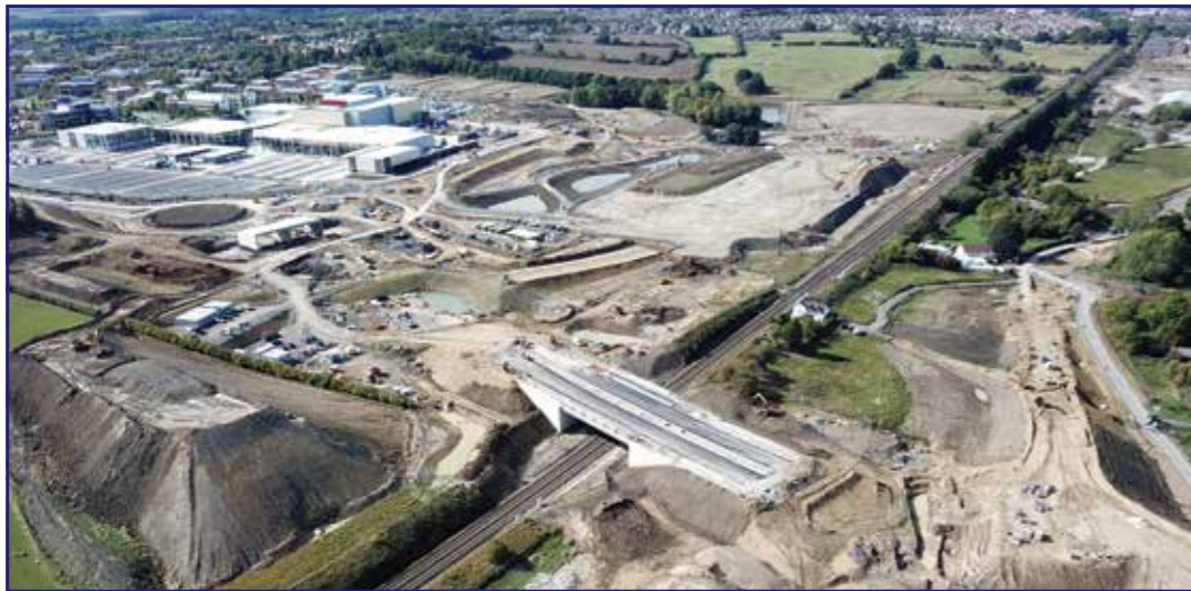
Early Stage Construction
