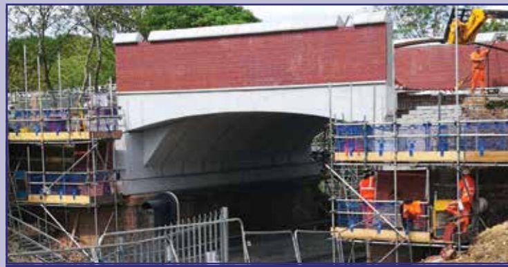
New Bridge Sits On The Old Victorian Abutments
