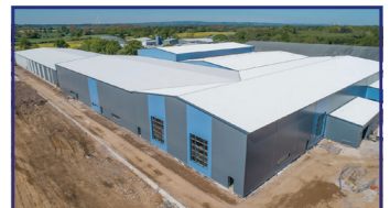
External view of the plant
