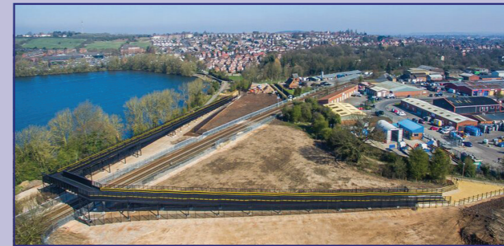
A birdseye view of the new King's Mill Lane crossing.
