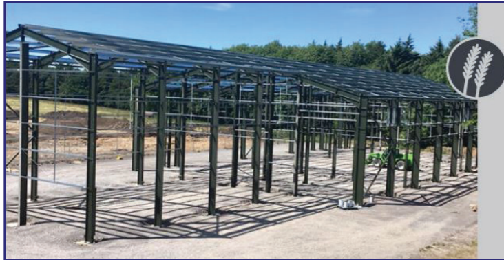
Wet grain intake building under construction
