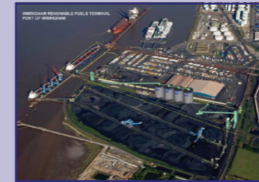
The vast IRFT with its huge machinery servicing requirement
