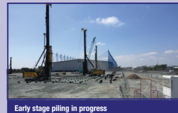
Early stage piling in progress
