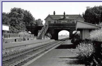
Former station at Irchester!
