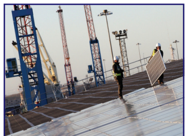
Installing the Solar Panels
