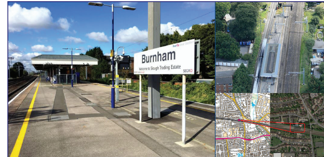
Burnham Station Access Improvements
