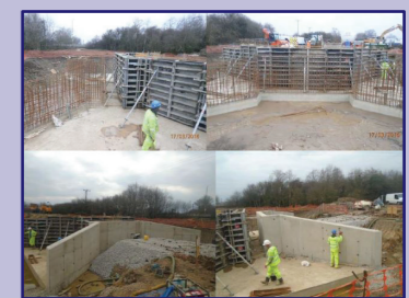
Some of the flow control structures being put in place
