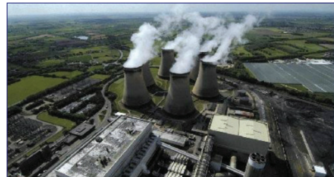
Drax Power Station
