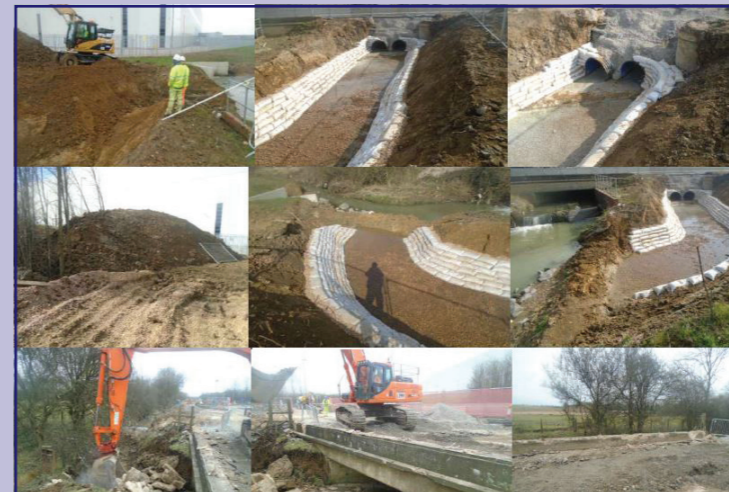
Work at Long Dole taking shape
