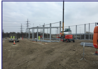
Work on Swift 13 Starts
