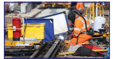
Working against the clock
