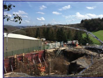
Concrete Piped Onto The Site
