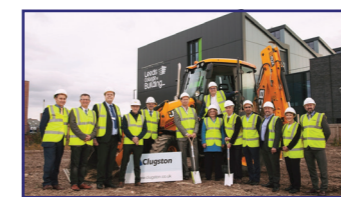
Clugston Construction on Phase 1
