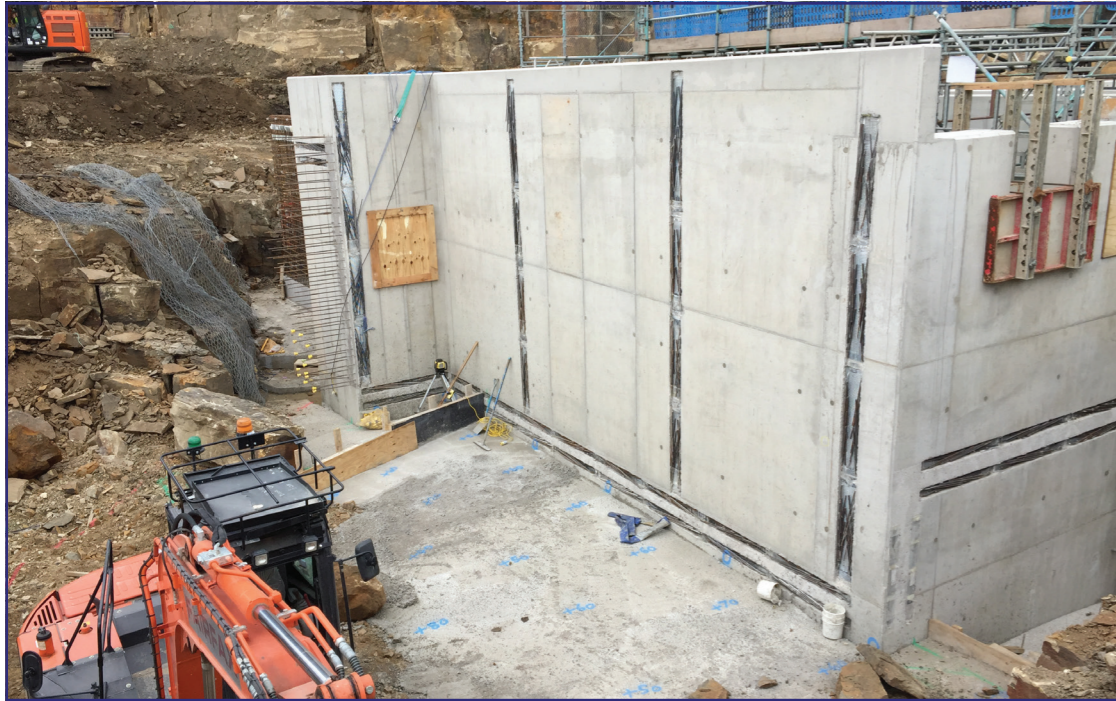
MIEX Facility Taking Shape
