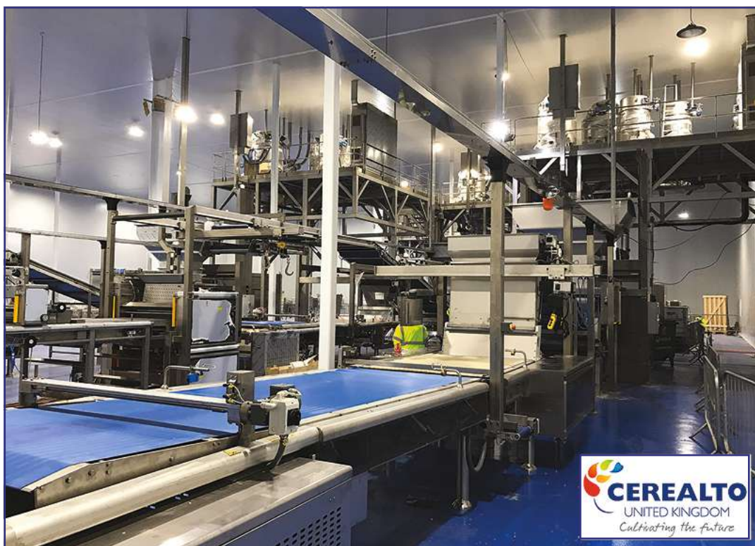
Cerealto Main Manufacturing Plant
