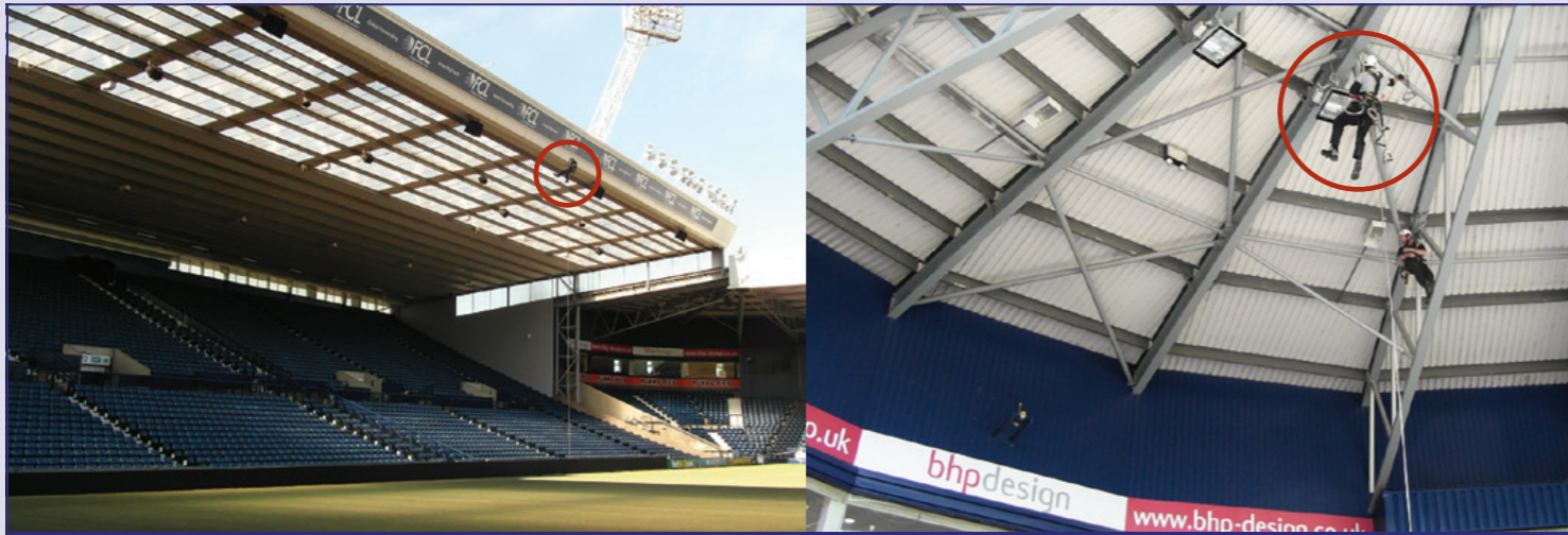
Inspection workers, circled - barely noticeable against the huge stand
