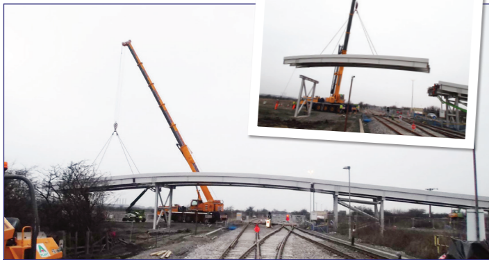
The over bridge taking shape
