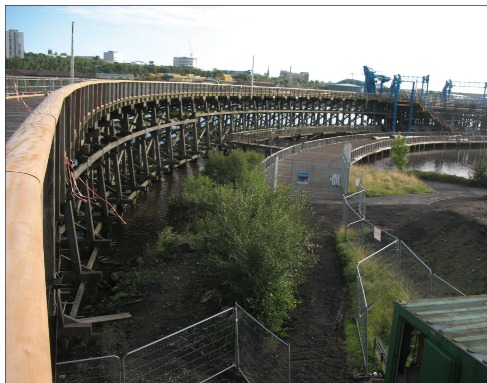
Dunston Staiths project: A view through the replacement handrail
