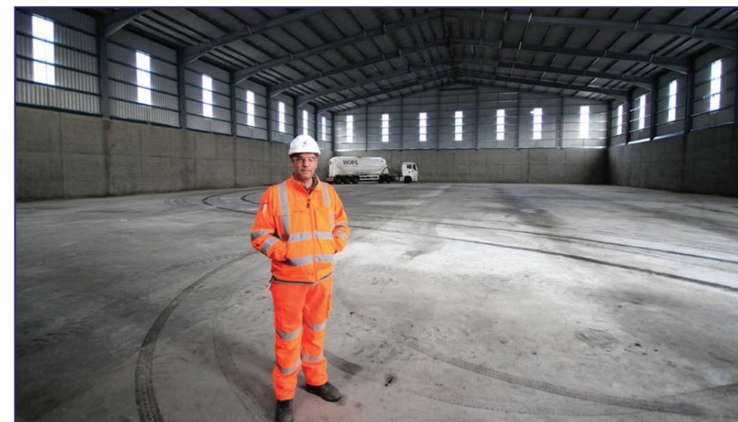
Hope Construction Materials' Industrial Director Ashley Bryan inside the new 20,000 tonne capacity clinker store
