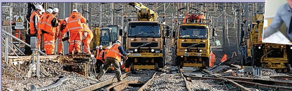
Electrification of the Midland Main Line
