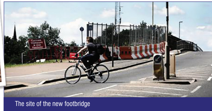
Work begins at Houghton Road
