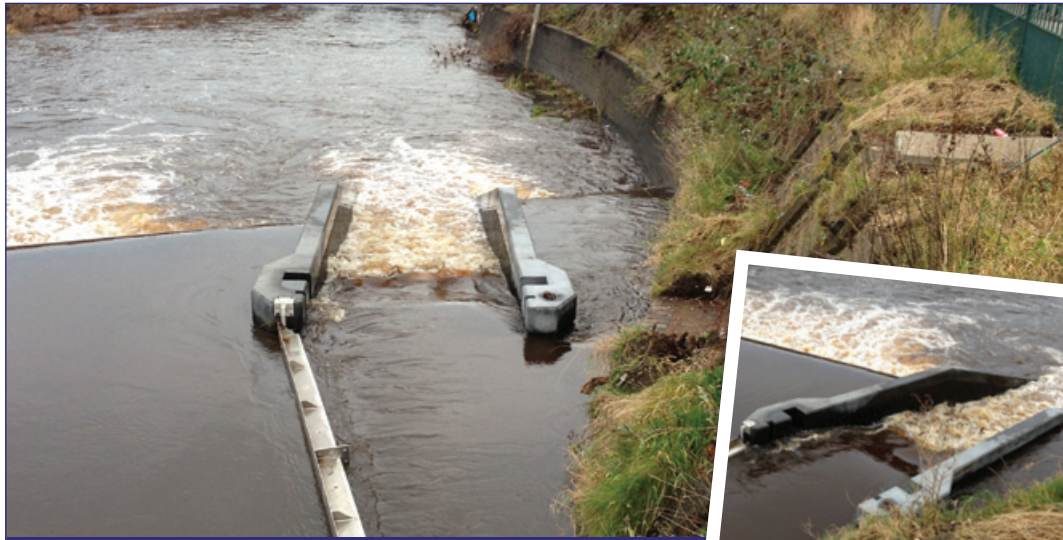
This and right: Making life easier for fish! The new fish pass
