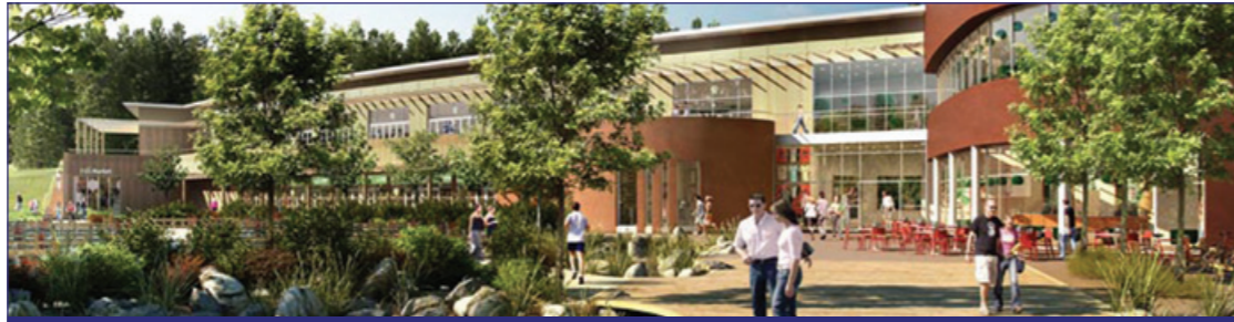
A Center Parcs Complex
