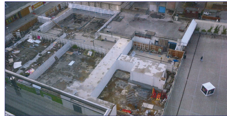
The site for the new retail, residential and hotel development
