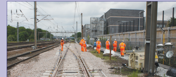
Work on the East Coast rail line
