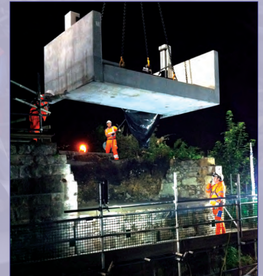
Working through the night on the underbridges
