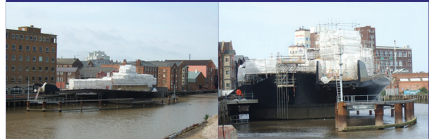
Building of the swing bridge and restaurant
