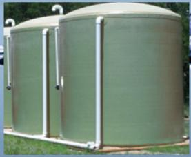
**Precast Concrete Unit Manufacturer - Nottinghamshire:** Considerable volumes of water are used for manufacturing precast concrete units for the construction industry, a large proportion being used for washing down; it is then discarded. Taking advantage of modernising their prestressing plant, a precast concrete manufacturer in the East Midlands installed a system to recycle water from their process, supplementing it with a rainwater harvesting system.
